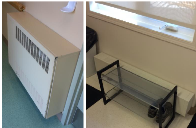
Figure 5: Hydronic Unit Heater (Left), Hydronic Baseboard Heater (Right)
