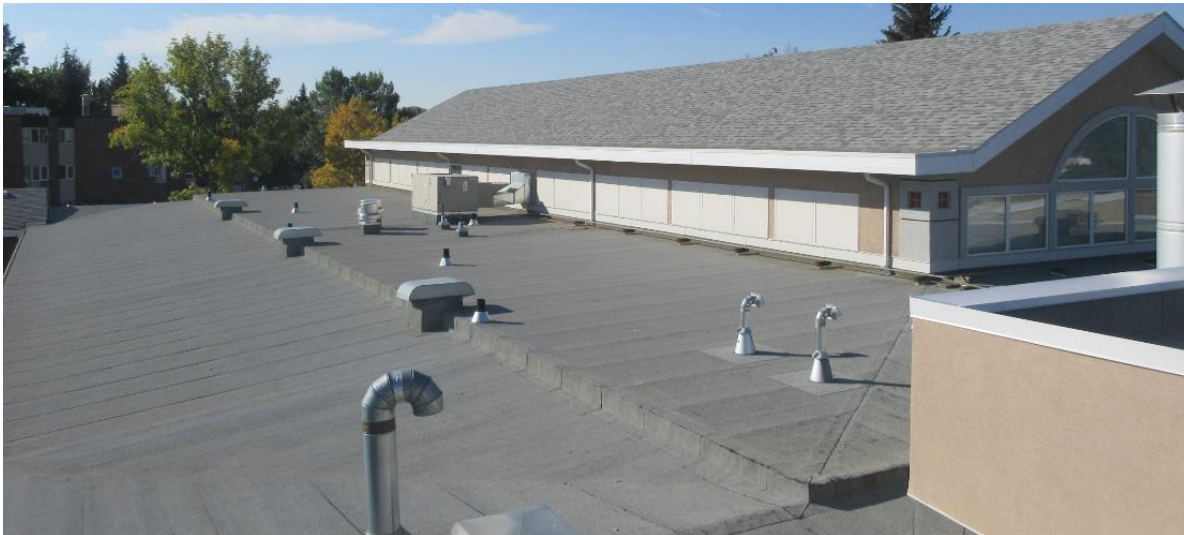
Figure 11: View of roof surface showing the Atrium clerestory windows
