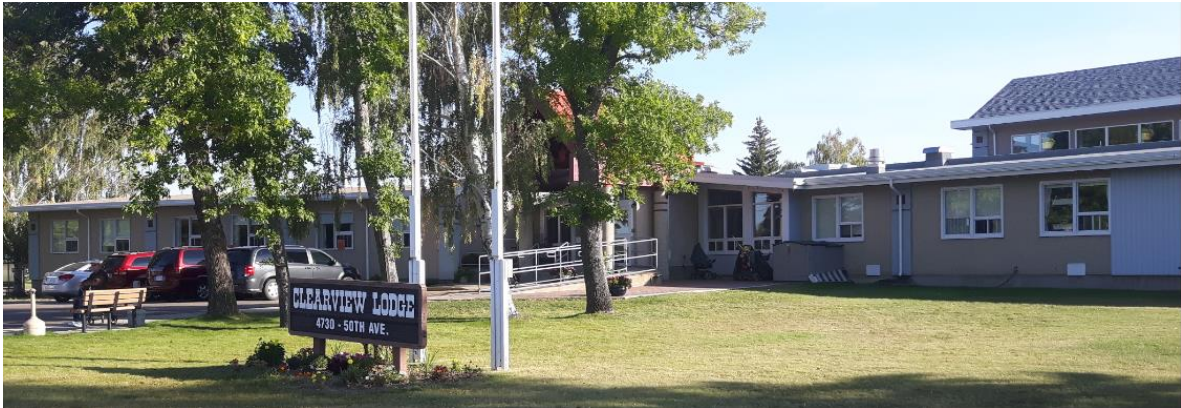
Figure 1: Clearview Lodge Front Main Entrance on the north wing
