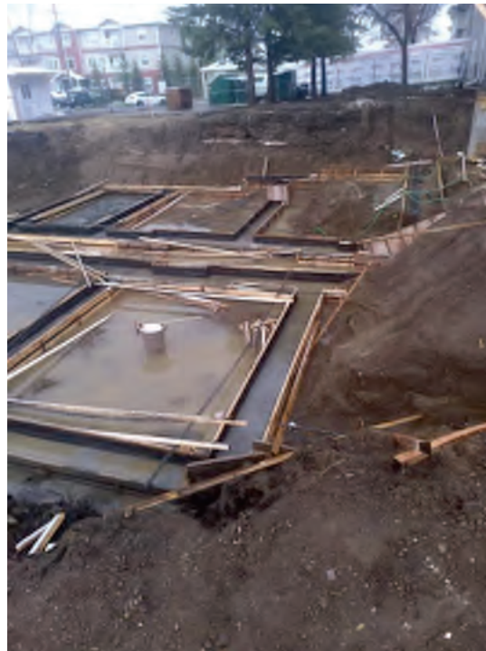
May 19th – Footing Status after Rain and Snow from the day before
