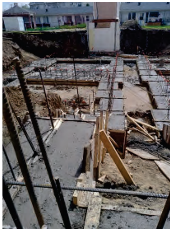
May 26 th – Strip Footings after the Concrete Pour
