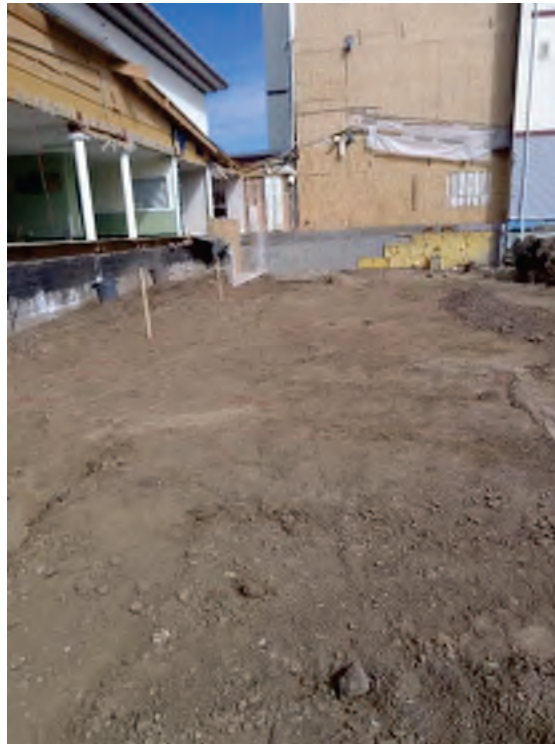
May4th: Excavation Progress at South of GL E and West of GL 7
