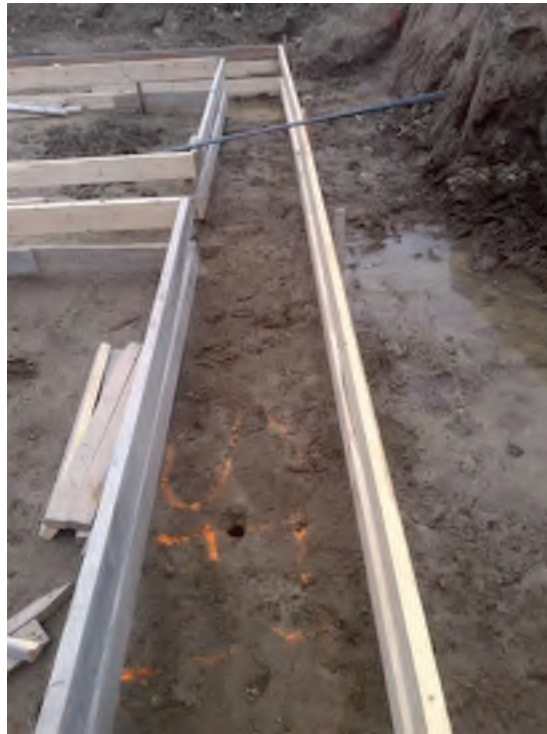
May 17th – Formwork of Strip Footings before Fillcrete Placement
