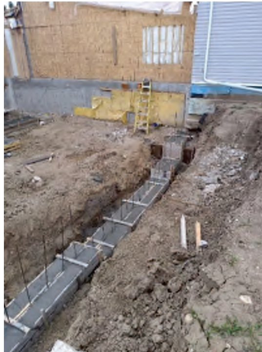
May 26 th – Strip Footings after Concrete Pour
