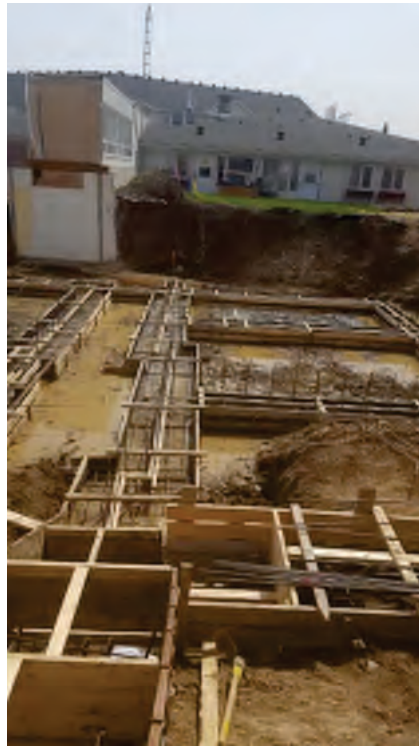
May 25 th – Progress on Footing Rebar Installation
