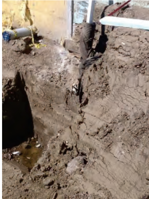
May4th: Excavation Progress by South Gridline E at GL 7
