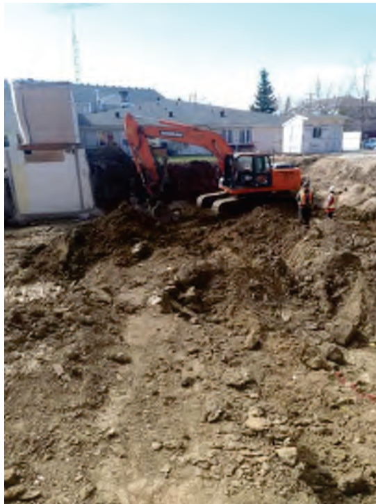
May 4 th - Excavation Progress North of Gridline A and between 7 & 10
