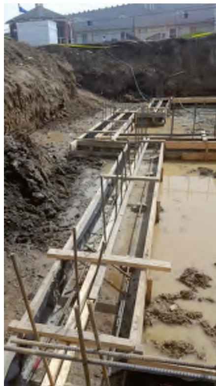
May 25 th – Progress on Footing Rebar Installation
