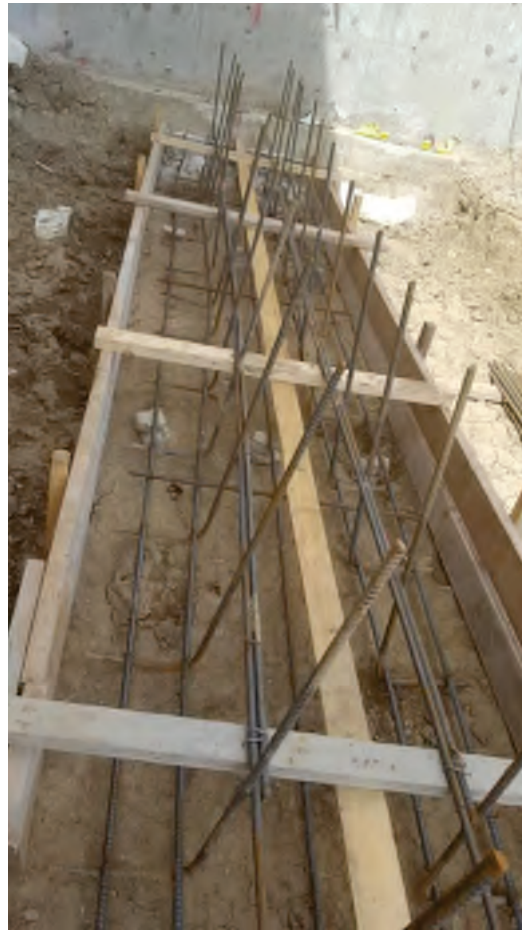
May 25 th – Progress on Concrete Reinforcement
