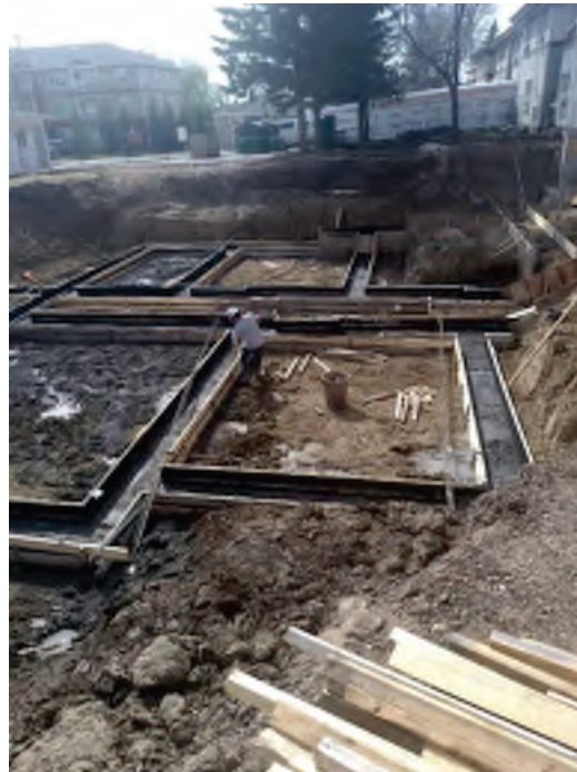
May 17th –Formwork of Strip Footings after Fillcrete has been placed to Prevent Muddy Conditions
