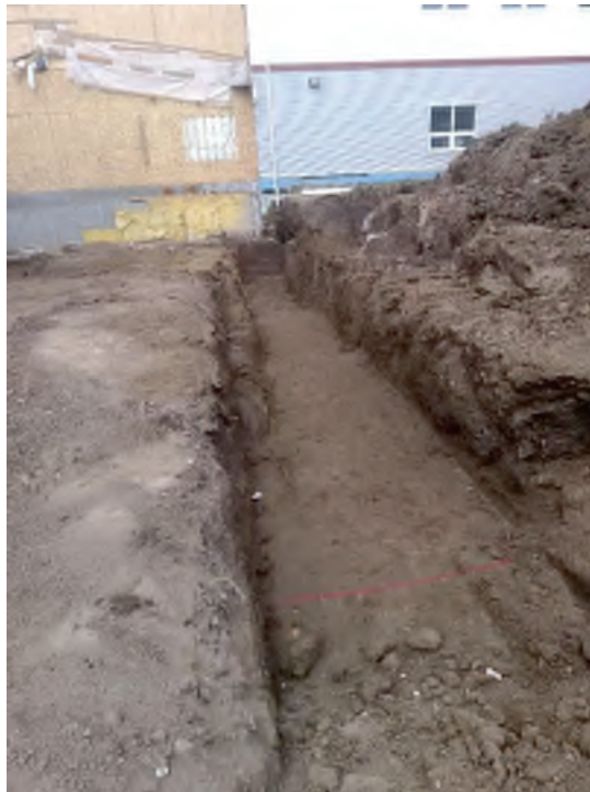
May4th: Excavation Progress along Gridline 7
