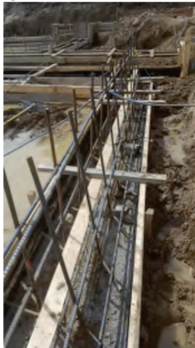
May 25 th – Progress on Footing Rebar Installation
