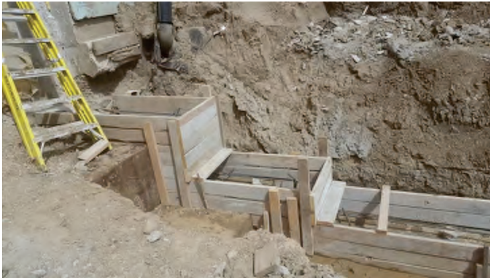
May 25 th – Progress on Formwork along South GL 7
