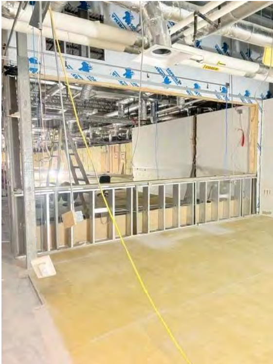
West Demo of Old Exterior Wall
