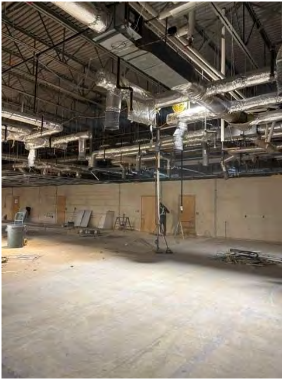
Demo North Area Up to Existing Corridor EP12H6
