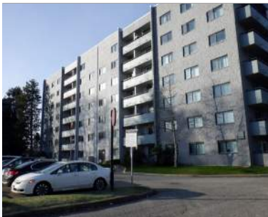
Rosewood Towers Richmond, BC Role: Superintendent
